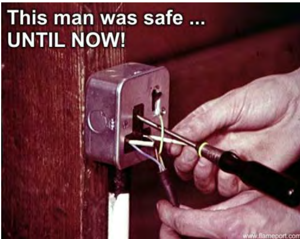
Fig 5.1.1.2: Example of a Potential Accident Area
