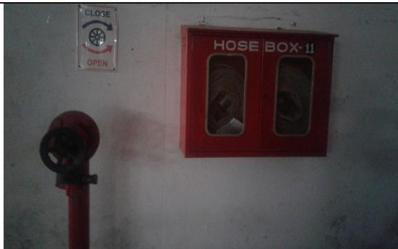
Fig 6.1.1.13: Water hydrant -For big fire
